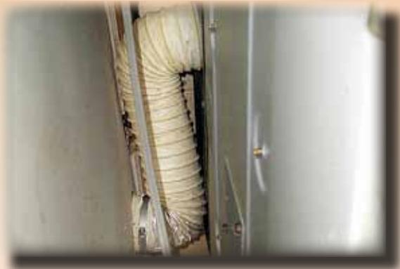
Answer: The hose is made of vinyl, which is susceptible to static charges; and the ridges, which are also on the inside of the hose, capture dust and lint, allowing for a dangerous buildup of flammable material. This is a fire waiting to happen. Dryers cause 1/3 of household fires, so if your hose looks like this, replace it immediately!
